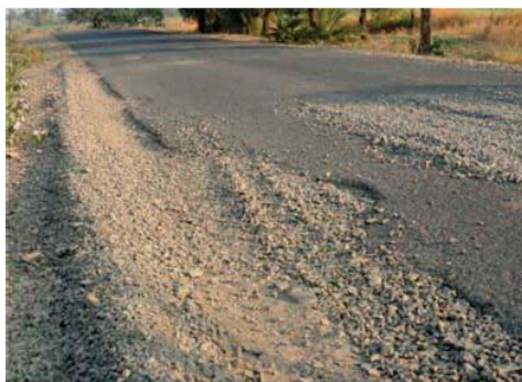
View of Basoda Sironj road under CRF
