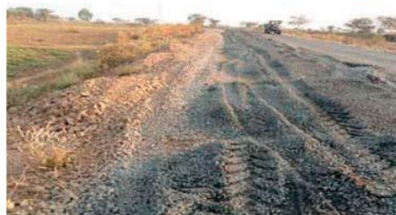
View of Basoda Sironj road under CRF
