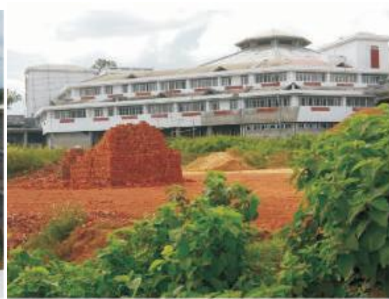
Construction of Assembly building scheduled in January 2009
